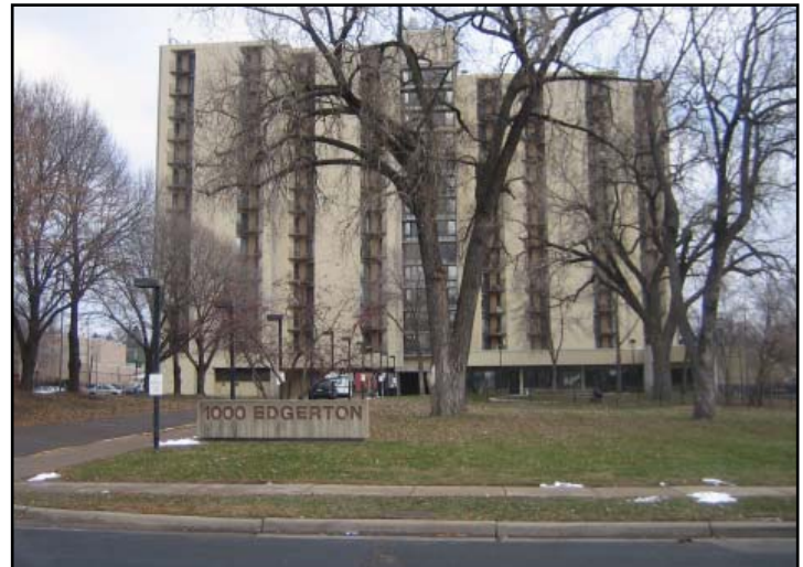
Figure 1: Site One; Public senior housing located in an established area of St. Paul, MN that did not receive funding from the Livable Communities Act's (LCA) grant-based programs.
