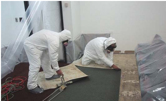
Carpet removal behind protective enclosure.
