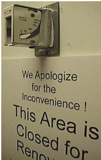
Construction barrier with manometer.
