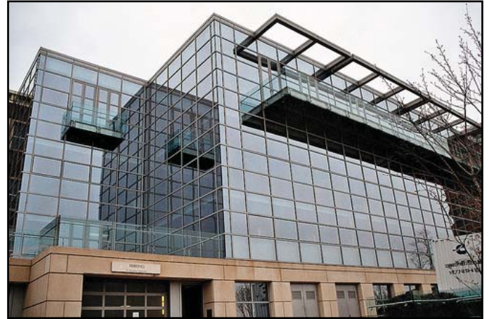
Figure 3: Example of a building with very large amounts of glass that likely has poor outdoor/indoor sound isolation. (Photo Copyright 2009 by idan586 and made available under an Attribution-Share Alike 2.0 license. http://www.flickr.com/photos/idan586/3552909176 )
