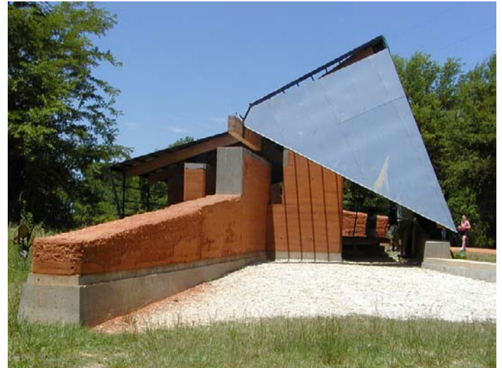
A chapel designed and built with Samuel Mockbee's students in the Rural Studio at Auburn University.
